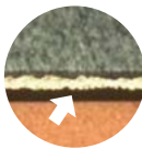
Remnants of plating
